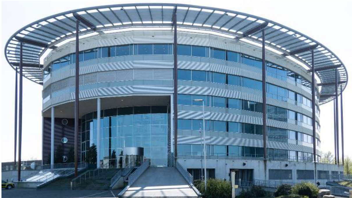
Figure 23: The HUB50, located centrally in The Netherlands (Nederlandse Politie, 2021d)
